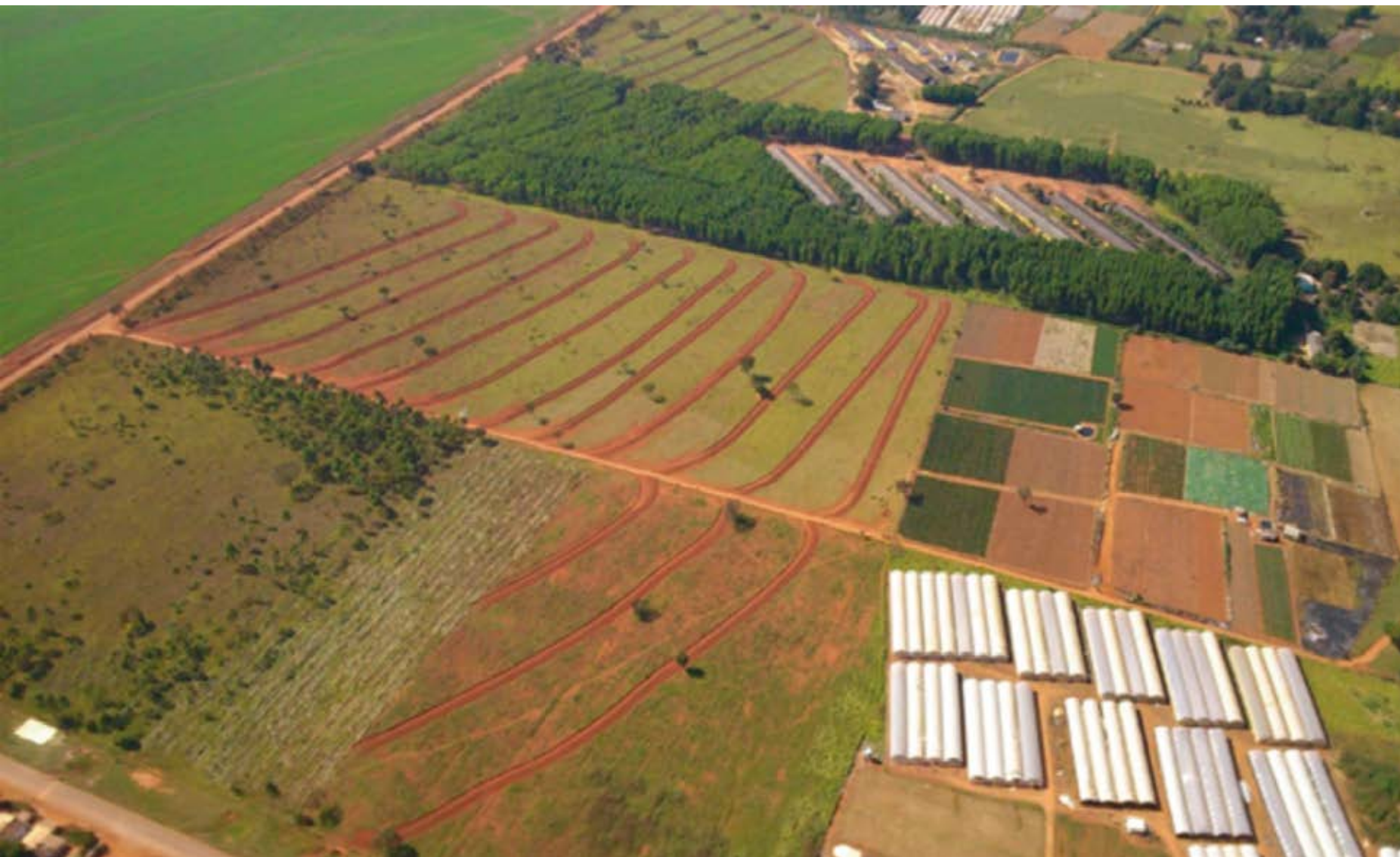
Figure 1. Aerial view after execution of level terracing Photo: ANA's Collection
